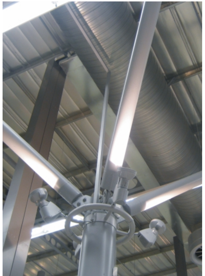
Special column luminaire c/w 4 x Cast A + D + J 150W MH
