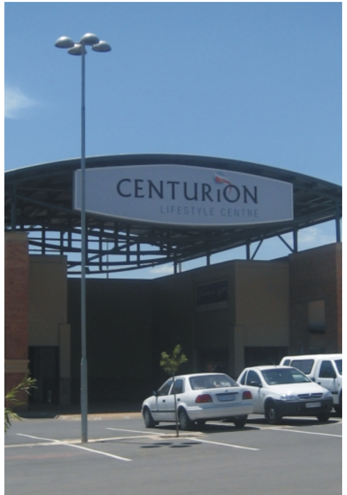
4 x Sun 150W MH luminaires on a 9m Galvanised Steel Pole
