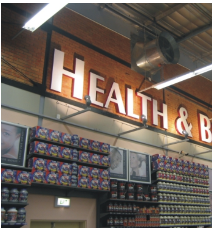
Cast A + C + J 150W MH on a special mounting track
