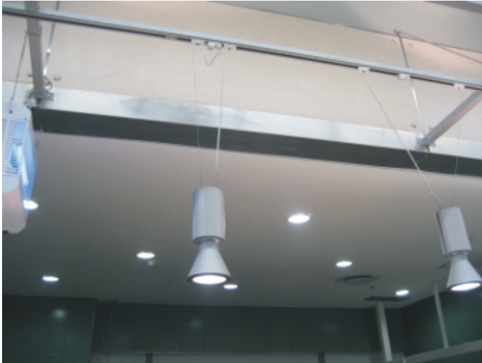
Vision E + N 70W MH track mounted with 2 x stainless steel cables
