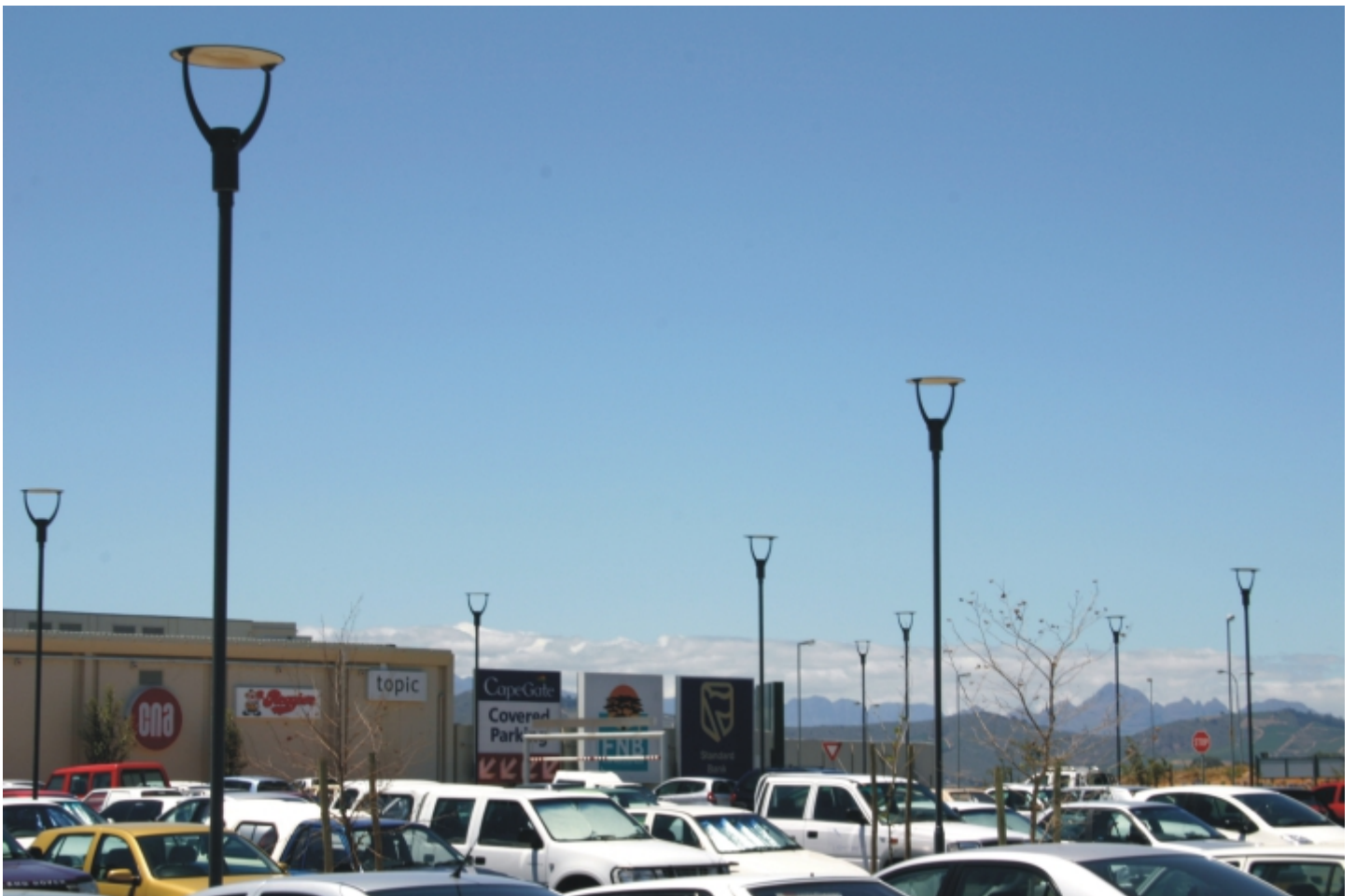
Saturn post top 150W MH on a 4m MH Pole
