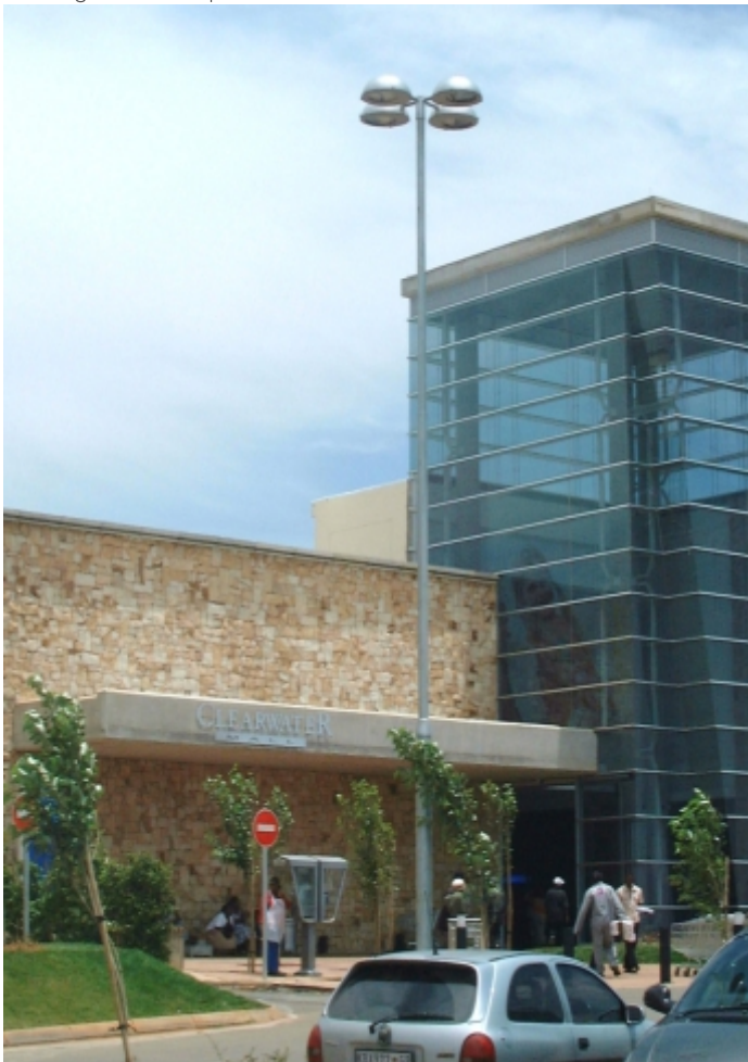
4 x side entry Sun fittings on a 9m galvanised steel pole
