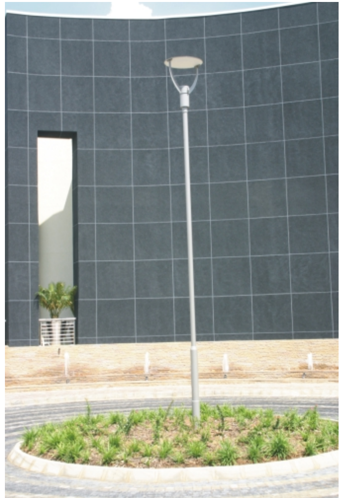
Saturn post top c/w 150W MH lamp on a 4m stepped pole
