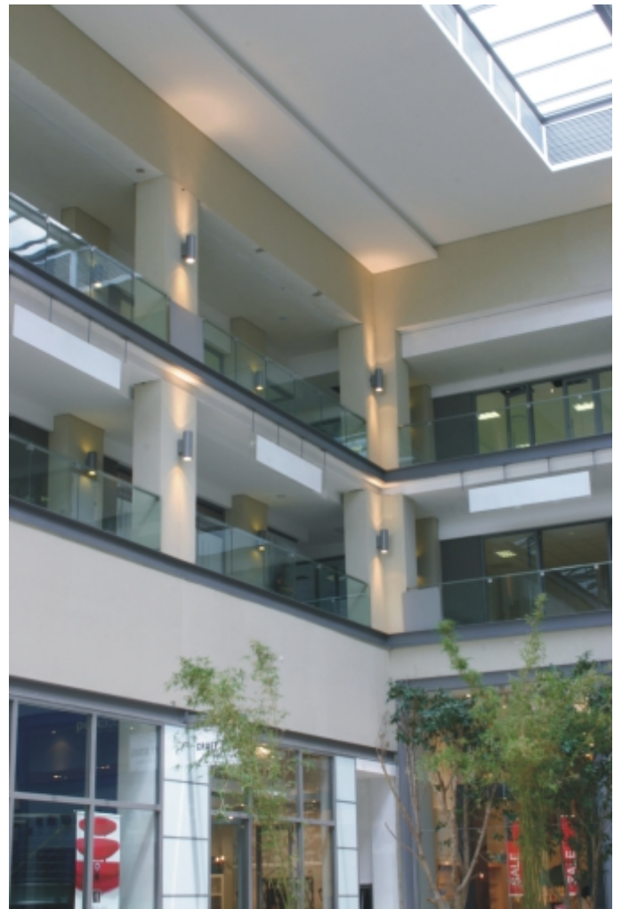
Beam up/down lighters c/w 20W Energy saver lamps
