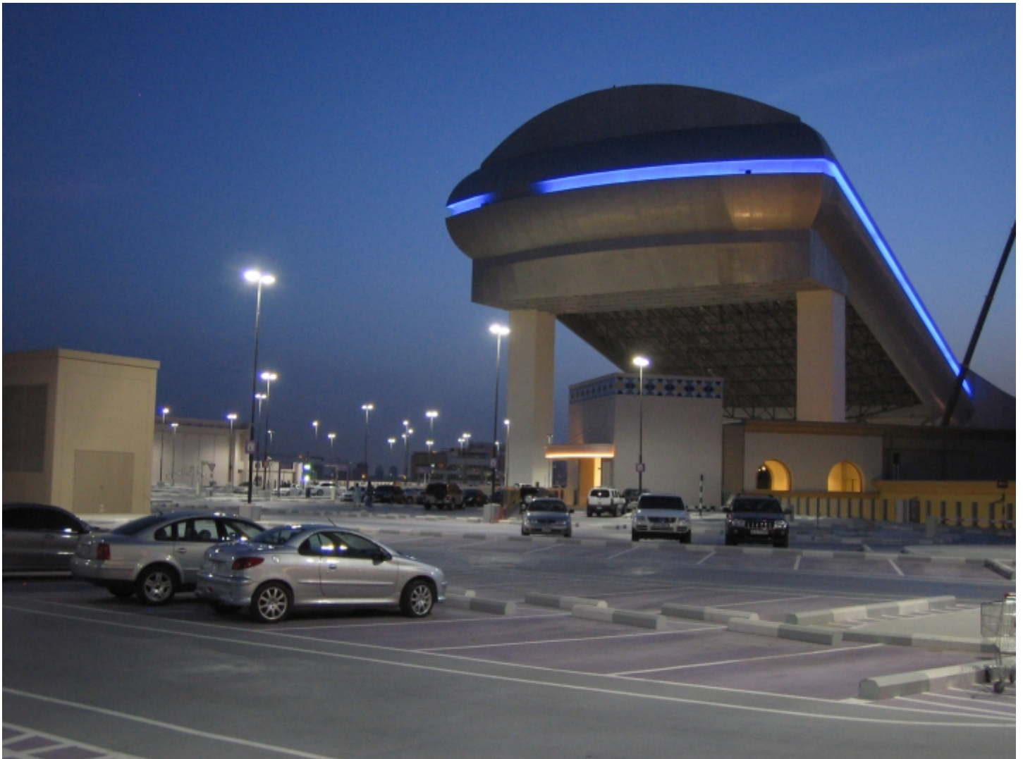
Pluto Double post top on a 9m galvanised steel split pole.
