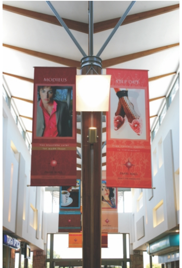
Wave 2 luminaires c/w 150W MH
