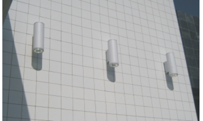
Beam up/down lighter 2 x 70W Metal Halide
