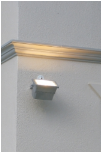
Gamma trunion mounted 70W Metal Halide
