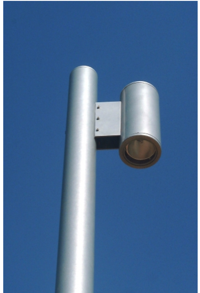
Beam post mounted down-lighter on a 4.5m 127mm diameter pole
