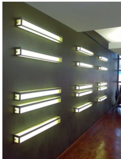
4m long special suspended fluorescent fitting complete with 3 x 58W lamp & ECG
