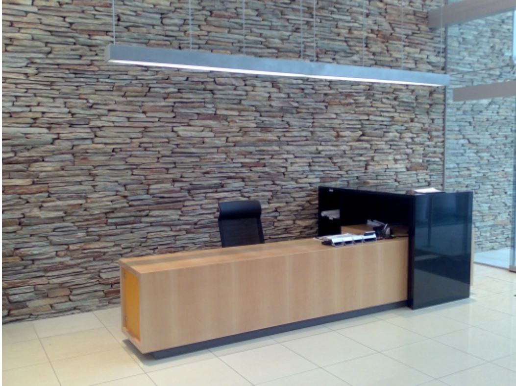
4m long special suspended fluorescent fitting complete with 3 x 58W lamp & ECG
