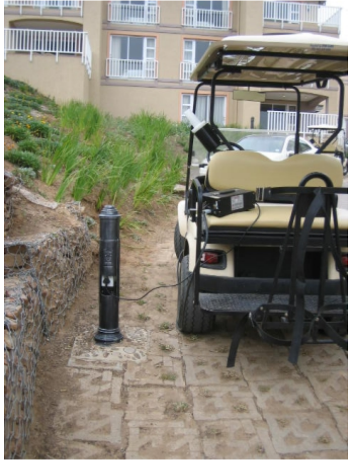
Special Helios Bollard adapted for charging golf carts
